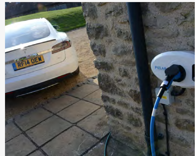
Figure 65: Example of off-street electric vehicle charging points.
