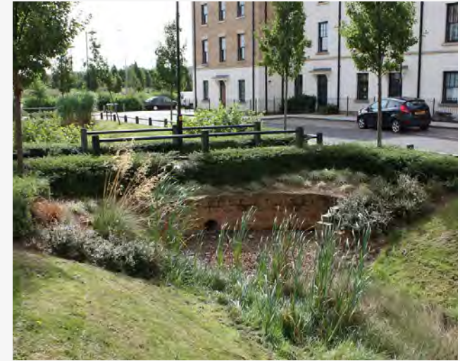
Figure 73: Example of swales check dam integrated with a crossing point, somewhere in UK.
