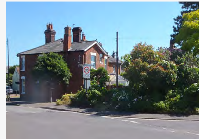
Figure 102: Local positive example of corner treatment where the building façades overlook the street on both sides, whilst hedges and trees create a curved boundary around the plot offering good visibility for pedestrians, Foundry Lane.
