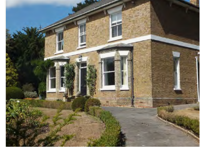
Figure 18: Victorian-style brick houses built by the Hunts Family in 1890s.
