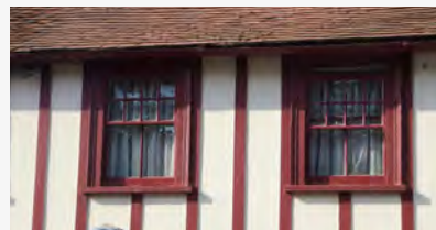
Casement windows with painted timber frame
