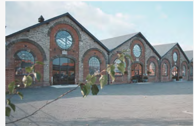
Figure 32: Central block of Atlas Works (Grade II listed) - redundant warehouses associated with Atlas Work Iron Foundry, retrofitted and refurbished as office spaces for local businesses. (Source: Historic England)
