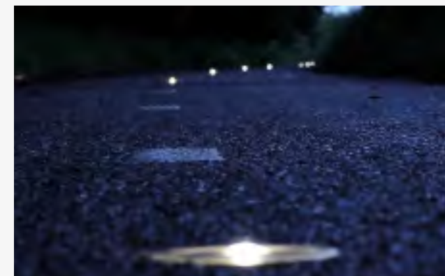
Figure 106: Example of a foot/cycle path which is lit by solar cat's-eye providing some light for pedestrian and cyclists without creating any disturbance to the nearby properties or unacceptable levels of light pollution.
