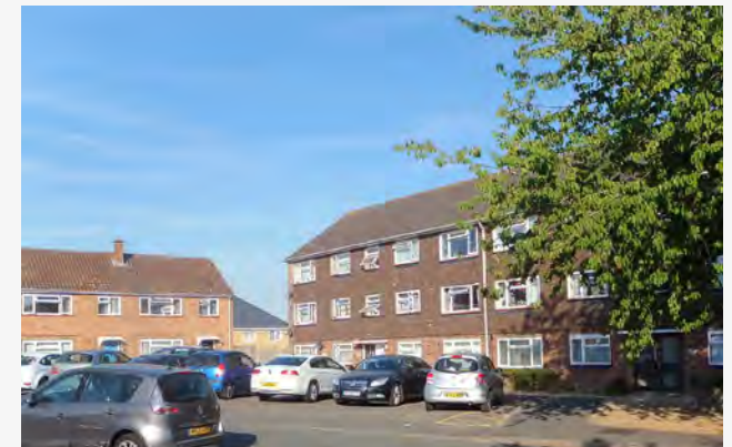
Figure 88: Flats on De Vere Road with green verges and parking court at front.
