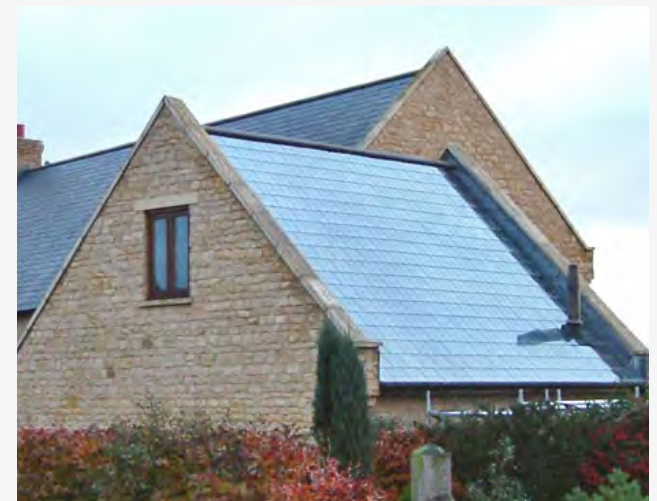
Figure 109: Positive example of implementing solar panels since the design stage.
