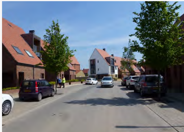
Figure 50: Secondary street with inset parking bays alternating with street trees on both sides of the street in Derwenthorpe York.
