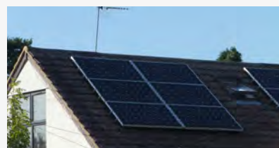
Rooftop solar panels
