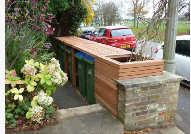
Figure 61: Example of wheelie bin storage for front gardens that include a green element to improve the aesthetics.
