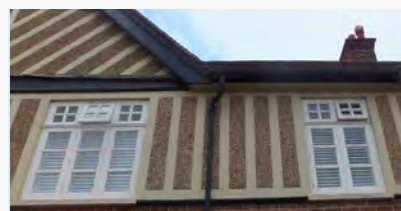
Modern casement windows
