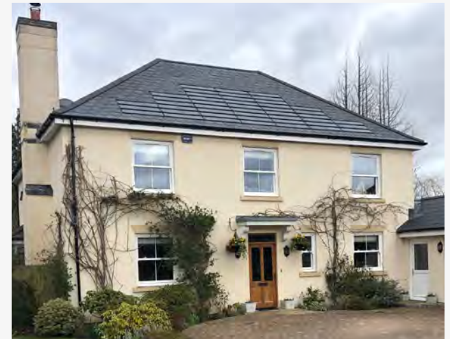
Figure 108: Use of shingle-like solar panels on a slate roof, with the design and colour of the solar panels matching those of the adjacent slate tiles.
