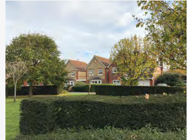
Figure 81: Positive example of new development where open space is equipped with trees and overlooked by properties, elsewhere in UK.
