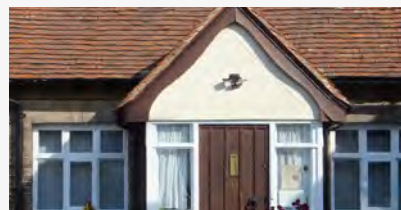
Gabled porch with timber door
