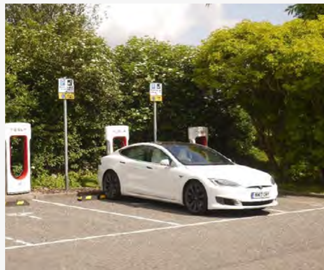
Figure 64: Example of electric vehicle charging points in a parking court.
